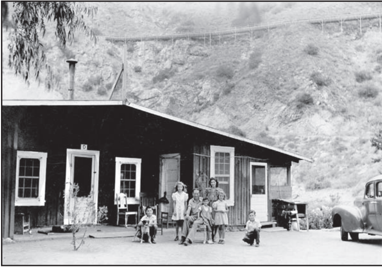
City House & Steel Flume Above
